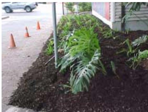
Plate 1. Application of a composted soil conditioner to a soil bed at The University of NSW.
