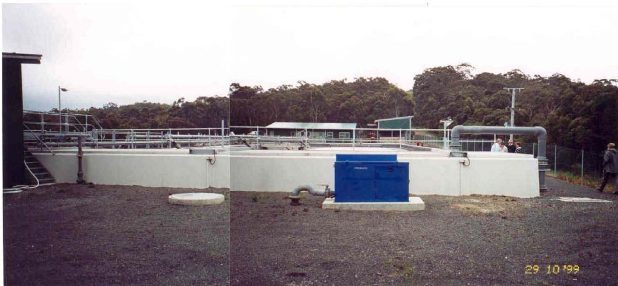
Figure 4.4.1.3: The completed treatment plant.
