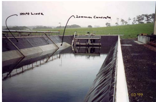
Figure 4.4.4.2: The completed treatment plant with additional remediation works.
