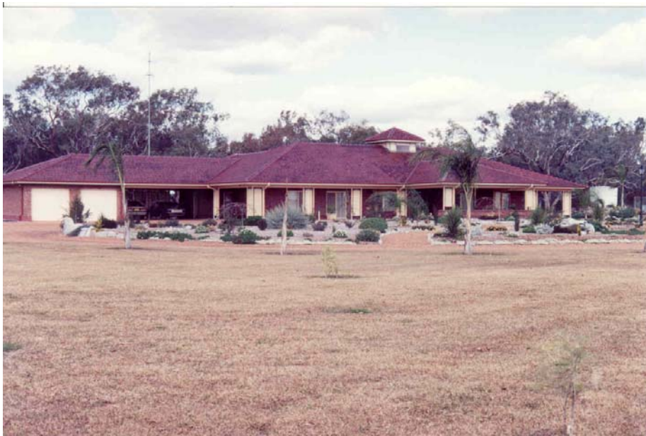
Figure 3.1: Overall view of house at Moree.
